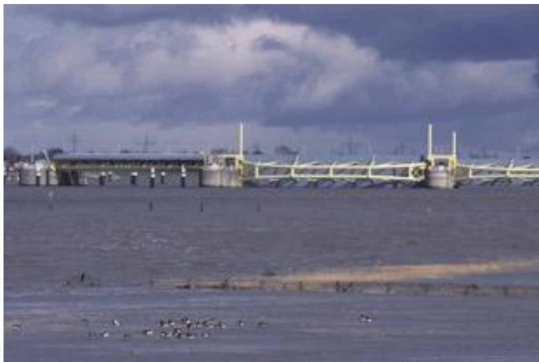
The Ems barrage near Gandersum is primarily used to dam up the Ems for ship transfers.
